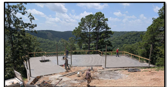
Wright Residence main floor concrete finishing Photo by G. Myers 7.20.26
