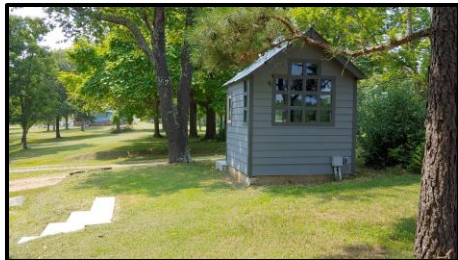
Rockspire's Pumphouse - back Photo by G. Myers 8.6.21
