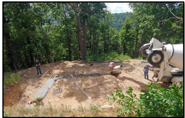
Mike Johnson observing concrete pour at homesites Photo by G. Myers 7.15.21
