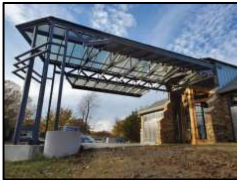
MobbyMac Carriage House canopy addition Photo by E. Chapman 11.4.20
