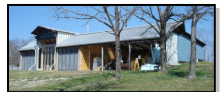
MobbyMac Carriage House progress Photo by G. Myers 3.24.11
