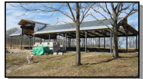
MobbyMac Carriage House progress Photo by G. Myers 1.29.06
